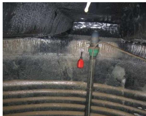
*The level switch (red) mounted inside the settlement tank.*
