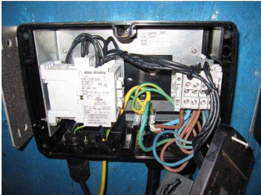
*Inside the Grundfos IO101 after the connections were in place. The white box on the left is the relay for automatic switching between solar and generator power.*
