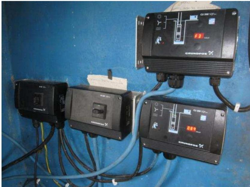
*The control boxes while operating. The panels are currently producing 0.89 kW.*
