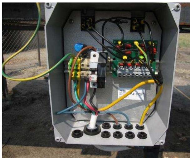
All the electrical protection provided by the panel control is provided by varistors, which do not protect against lightning which is the major threat to a solar powered system. It should therefore be considered to install some proper lightning protection in the future.
