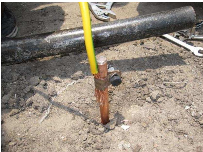
*The earth rod with an improvised clamp, it was forced into the ground so that it is no longer visible.*
