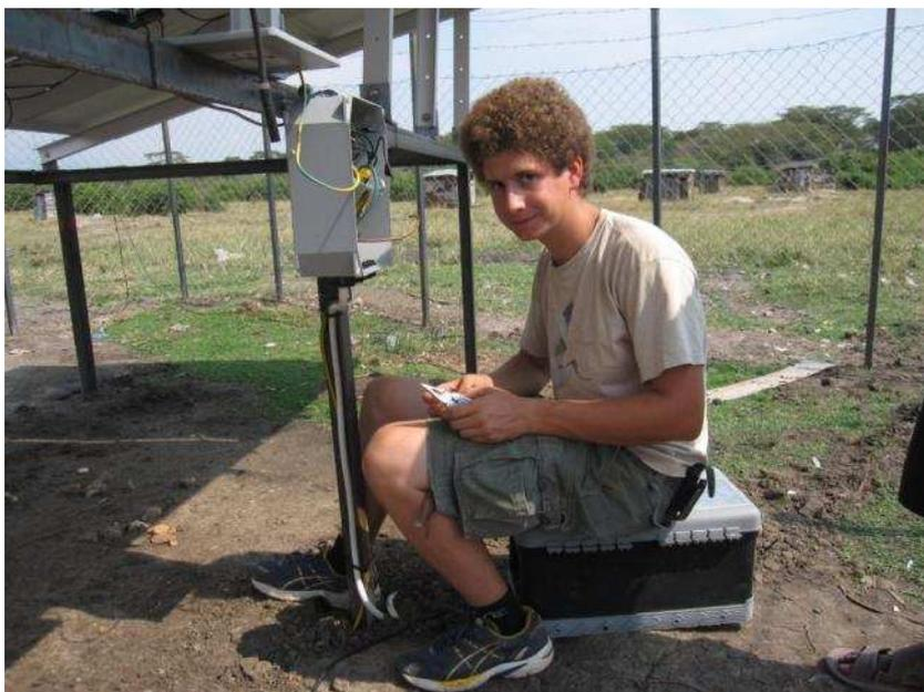
*Valentin Koestler having been responsible for the installation of the solar system is doing electrical connections in the control box for the solar panels.*
